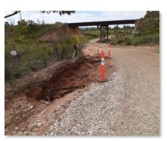
Picture 1 shows the loss of pavement materials as a result of sheetwash. Picture 2 shows destroyed and delaminated sealed surface and pavement damage and Picture 3 shows an example of shoulder destruction creating an immediate safety hazard for road users.
