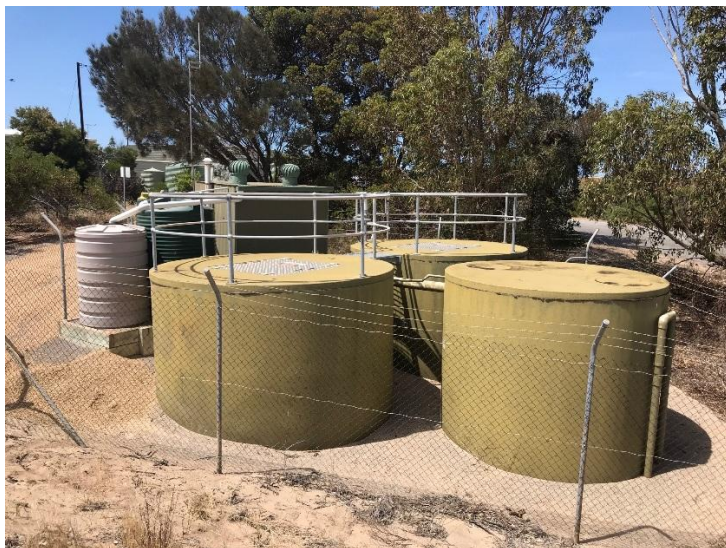
Figure 1 Rogues Gully wastewater treatment plant
