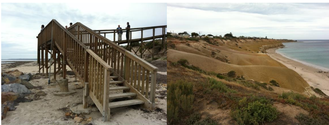
Figure 62: (Left) Christies Beach access stairs showing current erosion damage; and (Right) erosion damage along the southern edge of the Christies Beach foreshore (Photos: Adam Gray).
