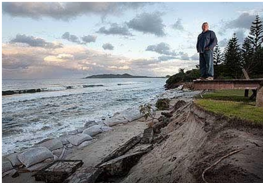
Figure 15: 'A cry for help... John Vaughan surveys his fast disappearing front lawn' (Source: Sydney Morning Herald, 2nd June 2009. Reproduced with permission from photographer Paul Harris).
