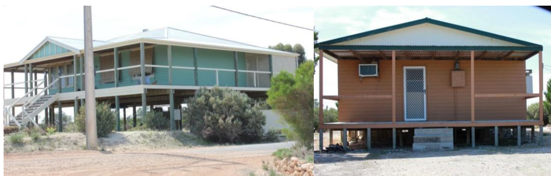
Figure 53: Example of Thompsons Beach dwellings raised above ground level (Photos: Jon Kellett).
