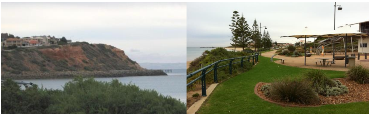
Figure 61: (Left) Existing rock defences at Witton Bluff (Photos: Jon Kellett); (right) the foreshore developments at Christies Beach (Photo: Adam Gray).
