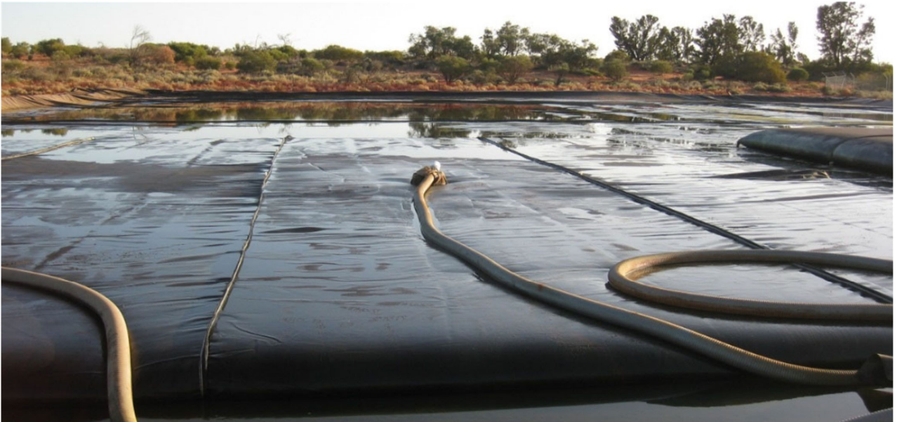
Figure 13 Geomembrane dewatering bag
