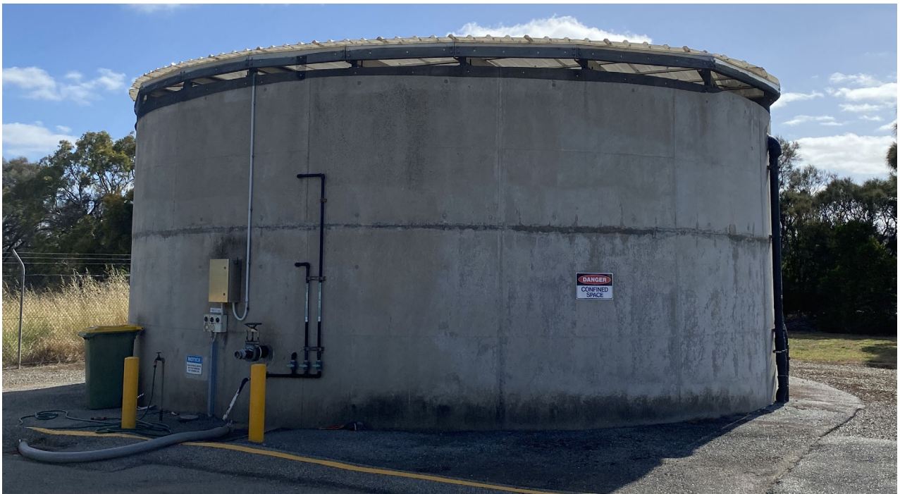
Figure 3 Willunga WWTP Gravity-thickened sludge tank
