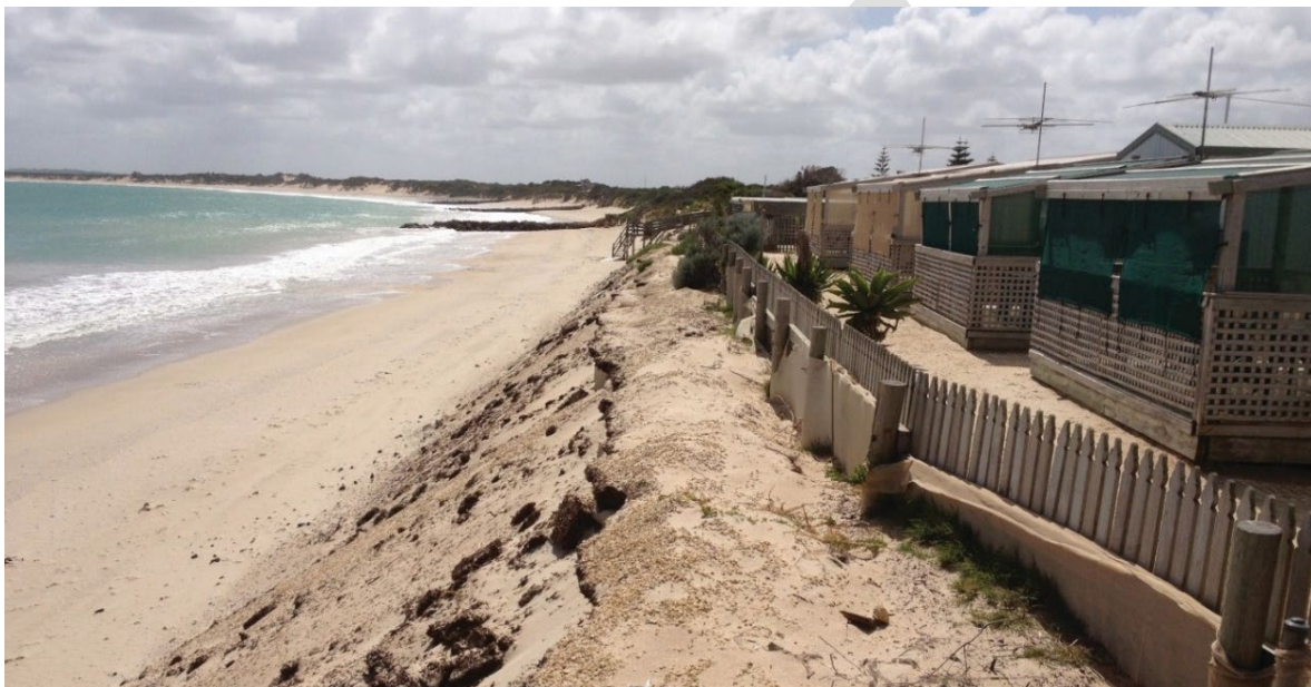
Figure 1: Picture showing impact of erosion on coastal community
