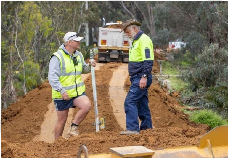
Figure 3: Council involvement in flood levees during River Murray Flood 2022
