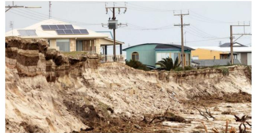
Storms swept away sand dunes and threatened houses at Wyomi Beach near Kingston in 2016. Photo: Kingston District Council
